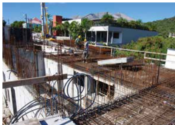
Construction parasismique © MEDDE
